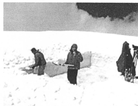
Clearing the site for work
