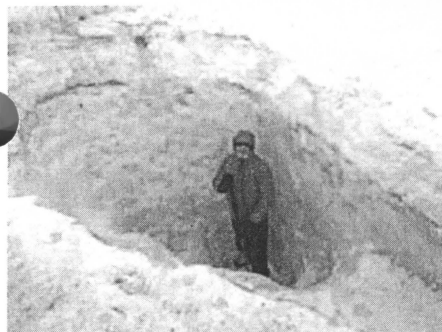
Randall cutting the hole
